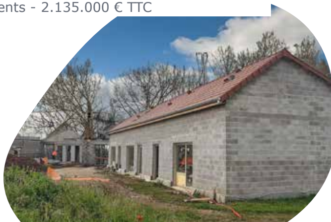
Oucques – ESAT Construction de 20 logements-foyer 2.883.000 € TTC
